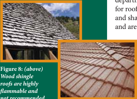
Figure 9: (above right) Class A roofing materials including tile, clay, concrete, slate and asphalt shingles are fire-resistant options. Photo: CSFS
